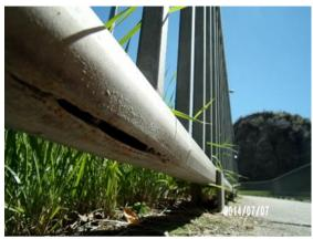
Thereafter, moisture accumulates faster than it can escape and builds up in non-draining areas, possibly over several cold weather periods/years. The HSS member finally cracks and releases the moisture. Also, corrosion build-up is taking place inside the HSS contributing to strength loss. Corrosion filled moisture may react differently when frozen than straight water in a clean test sample, suggests the reporter. Heat (direct sun exposure up to 70°C) may also affect the area in some way.
