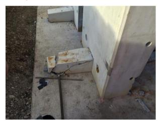
The use of shims, particularly under the body of the unit (as well as the feet) raised concerns regarding the temporary stability of the units prior to their incorporation into the parent structure. After an investigation, the following measures were taken:
